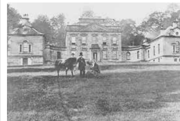
1860s Photograph showing East front of the house
