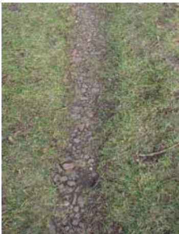
C05 East drive, section of old surface
