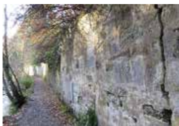
B28 Riverside path retaining wall and riverbank
