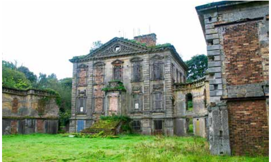
B01 Mavisbank House, east front and part of north pavilion seen from the north
