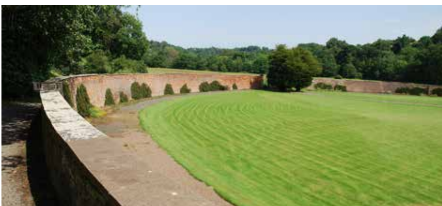
B04 Walled garden, north quadrant centre left being part of the original circle of walls; east quadrant (distant right) with windows to former cricket pavilion (B09)
