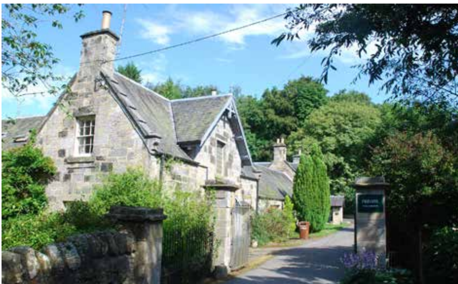
B07 Dairy, including south lodge and gate-piers
